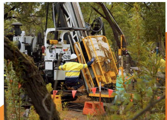
Small track mounted rigs are used to minimise impact.
